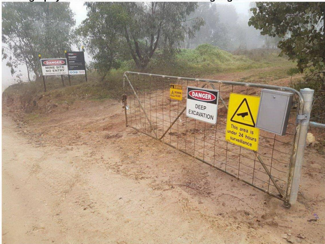
Photography 1: Locked Entrance Gate with Signage
